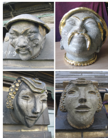
Figure 14. Top: "Chinaman" sculpture removed from the facade and renovated in the laboratory. Bottom: in situ renovated sculpture of a woman. Photo by M. Gašior
