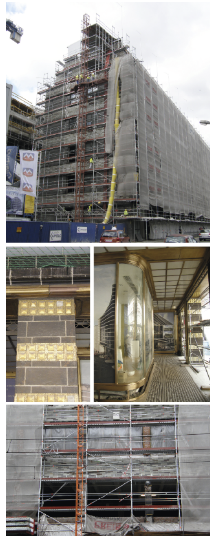
Figure 9. Conservation works at the facade of Renoma department store. Top: best preserved eastern part of the building. Middle left: pillar faced with ceramic tiles and gold plated mosaic. Middle right: renovation of brass display windows and of the backlit grate. Bottom: severely damaged western facade with renovated parapet walls. As in 2008. Photo by P. Kirschke
