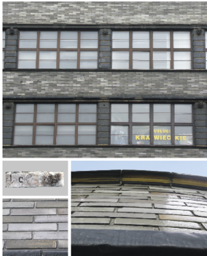
Figure 5. 2006 condition of facade designed in 1930 by Herman Dernburg. Top: relatively well preserved central part of the northern facade. Middle: ceramic tile showing the mark of Richard Blumenfeld Velten AG brickyard. Bottom right: attic wall at the rounded corner from Świdnicka street side; the sill tiles were bent before burning. Bottom left: fragment of flat wall faced with small size tiles, some of which were gold plated. Photo by P. Kirschke, 2006-2007
